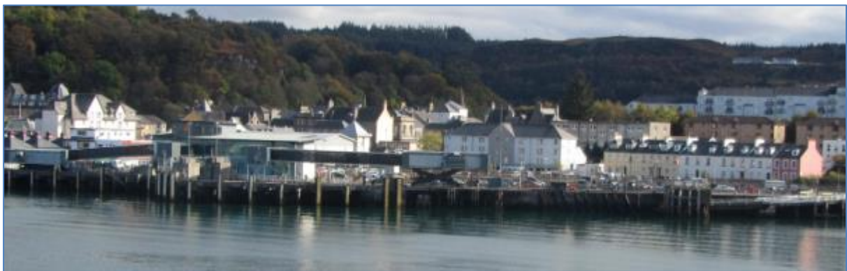
Figure 9: Railway Jetty showing the two RoRo berths.
