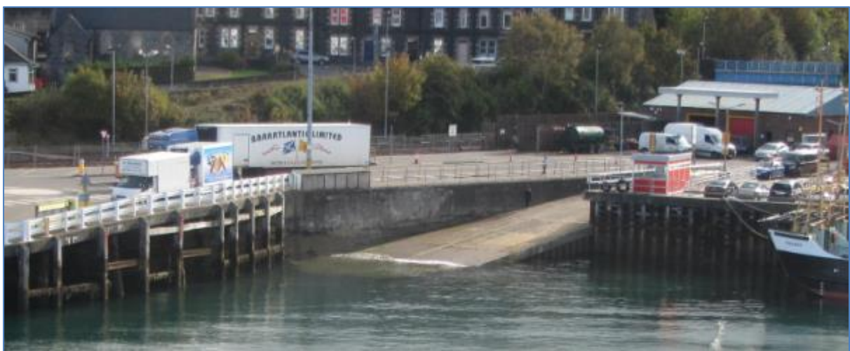
Figure 10: Slipway for small ferries.
